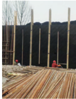
Phase 1 construction of logistic centre
